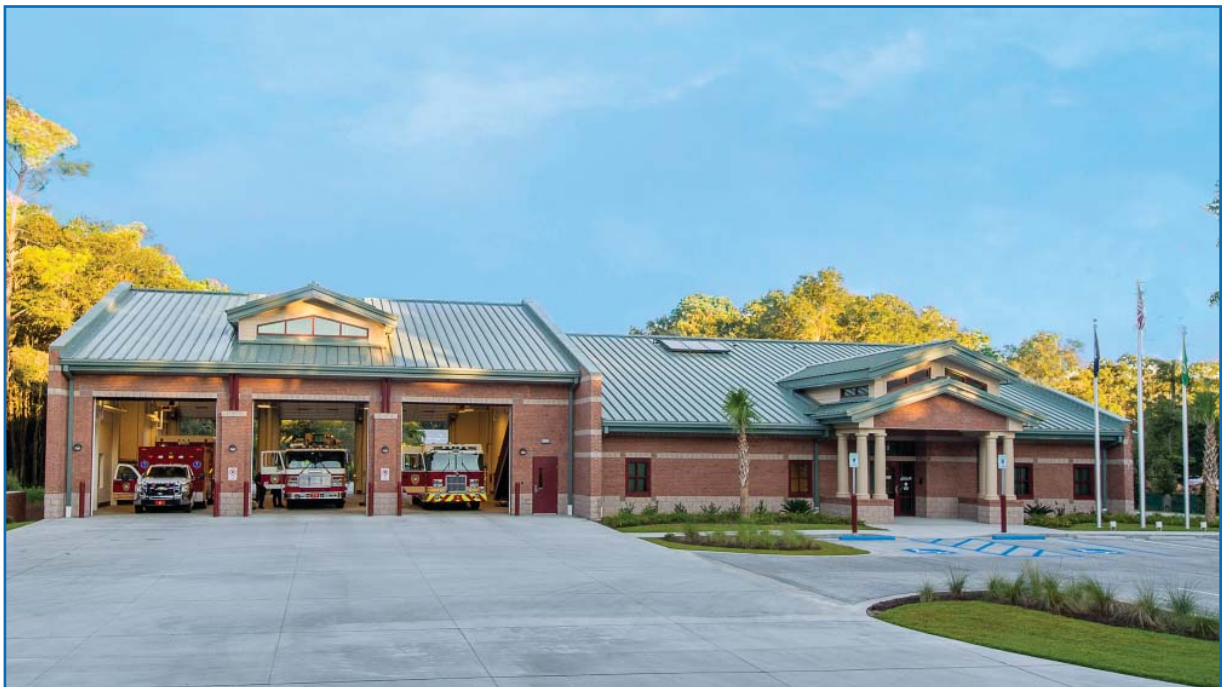
Hilton Head Island SubStation: Example of Pre-Engineered Construction
