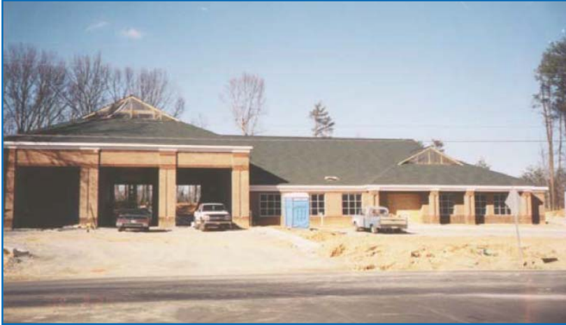
Conventional Construction During Construction
