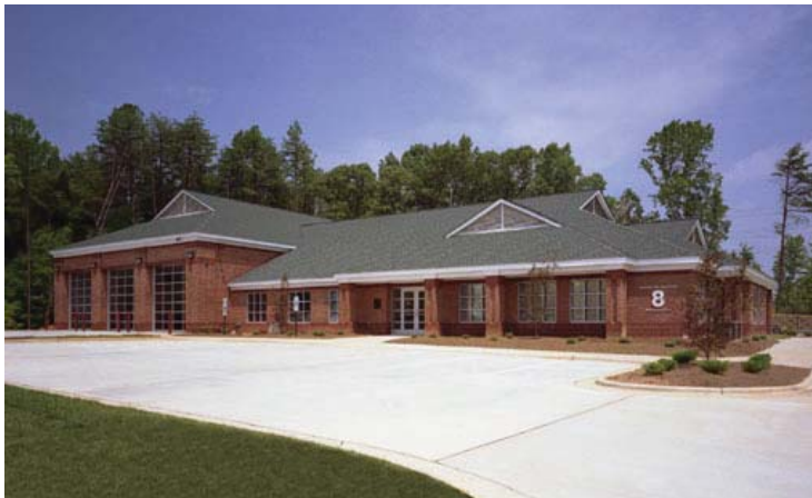
City of Gastonia Prototype Sub Station: Example of Conventional Construction
