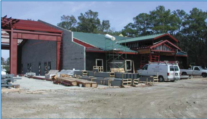
Hilton Head Island SubStation: Pre-Engineered Under Construction
