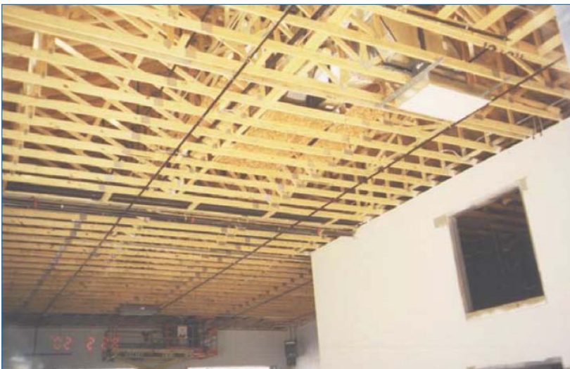
Example of Conventional Construction Wood Roof Trusses
